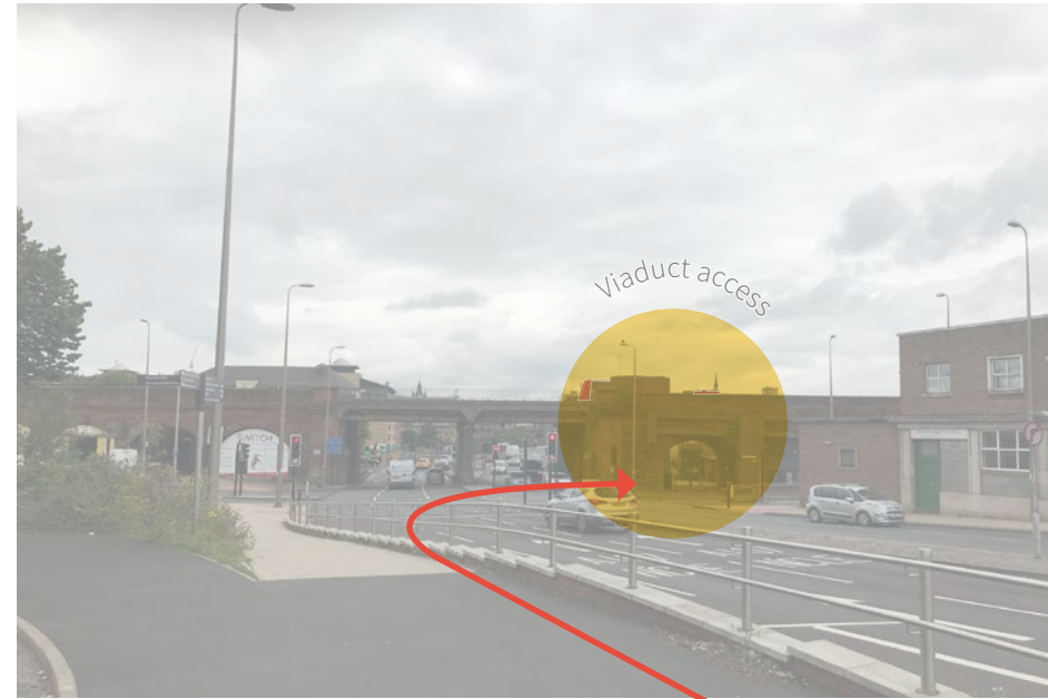
2 View from Nelson Street, facing towards the viaduct
