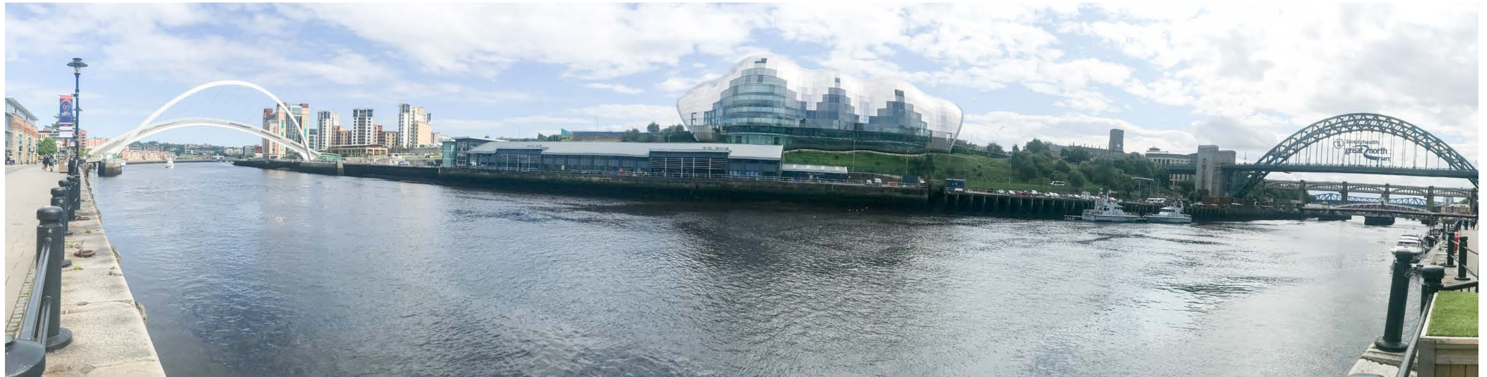
VIEW FROM HADRIAN'S WAY FACING SOUTH TOWARDS THE FRAMEWORK AREA
