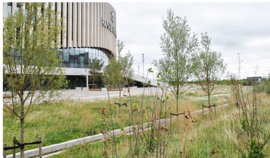
◀ Softening public realm along Oakwellgate and to the west of Sage Gateshead
